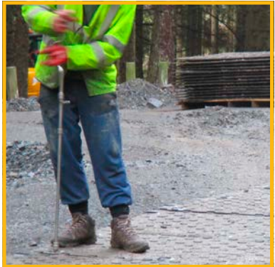
Install bolts carefully to avoid cross threading
